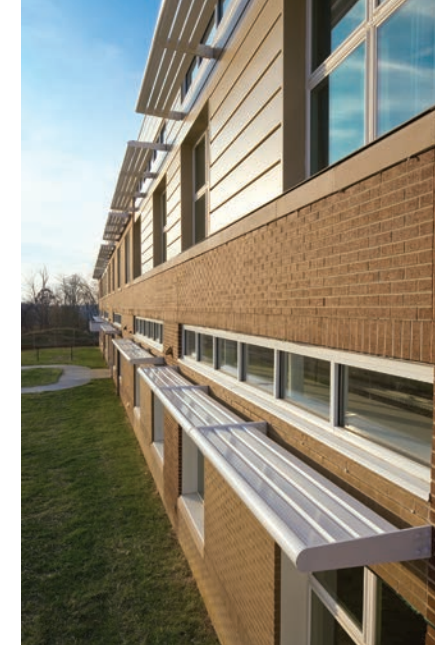
The south side of the building has exterior lightselves to direct sunlight further into the classroom.
