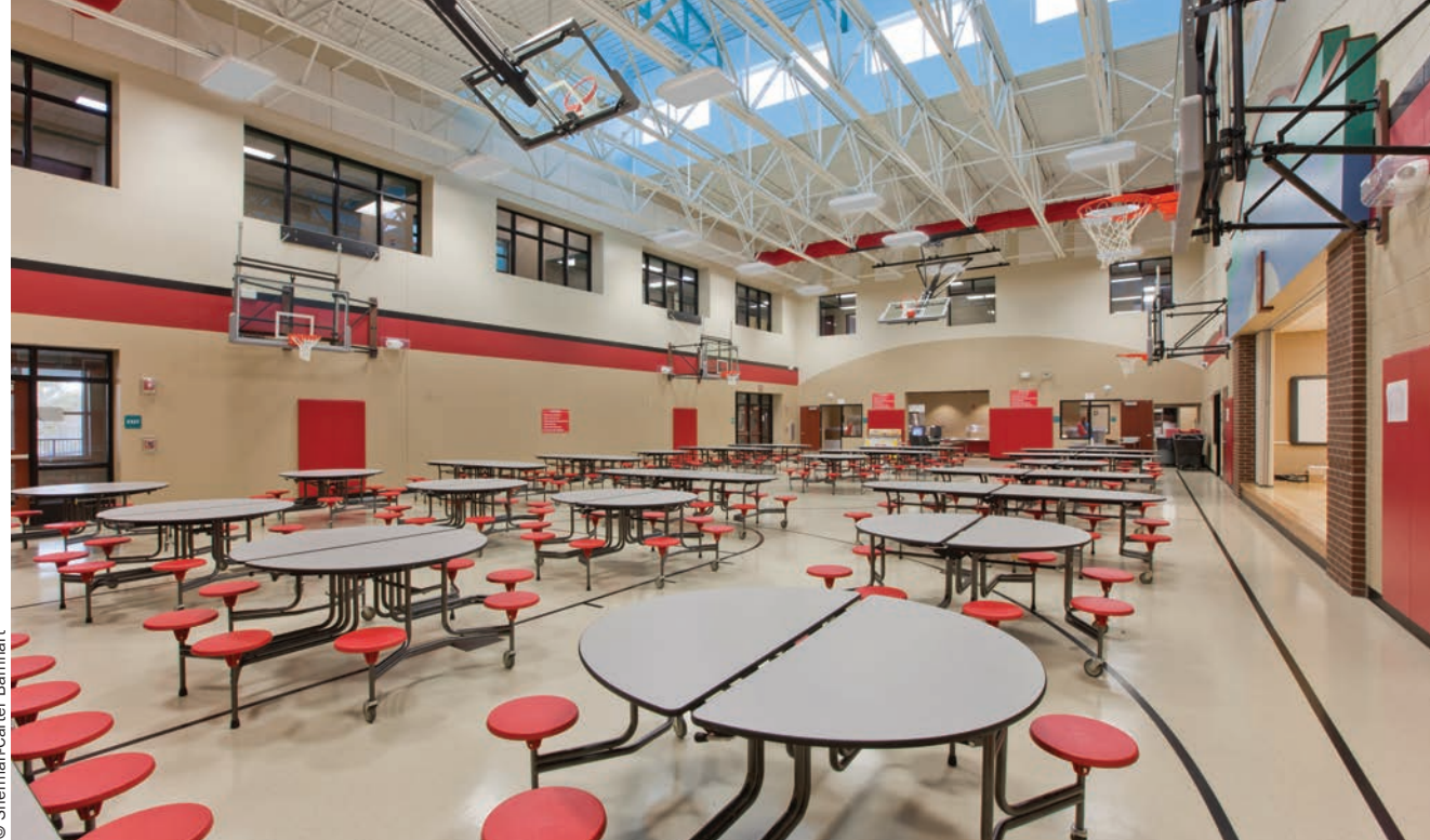
The gymnasium serves as gym and cafeteria. The cafeteria setup is pictured here. The clerestory windows that form the spine of the building and admit daylight into the main hall and gymnasium/cafeteria can be seen at the top of the photo. None of the overhead lights were on when this picture was taken.
