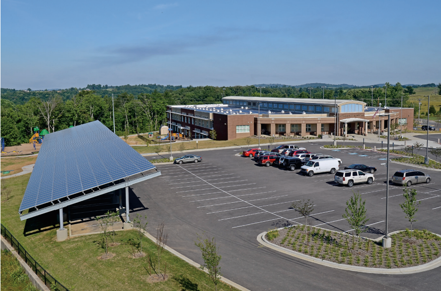
Above A 140 kW crystalline array mounted on a parking shade structure and a 208 kW thin-film rooftop array provide the school's renewable energy.
